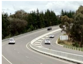
Central median barrier
