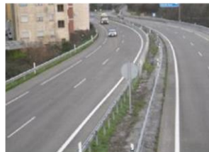
Duplication with median barrier
