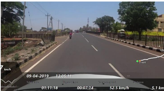
Poor condition of footpath and broken pedestrian fence Km 5.1, SH-20
