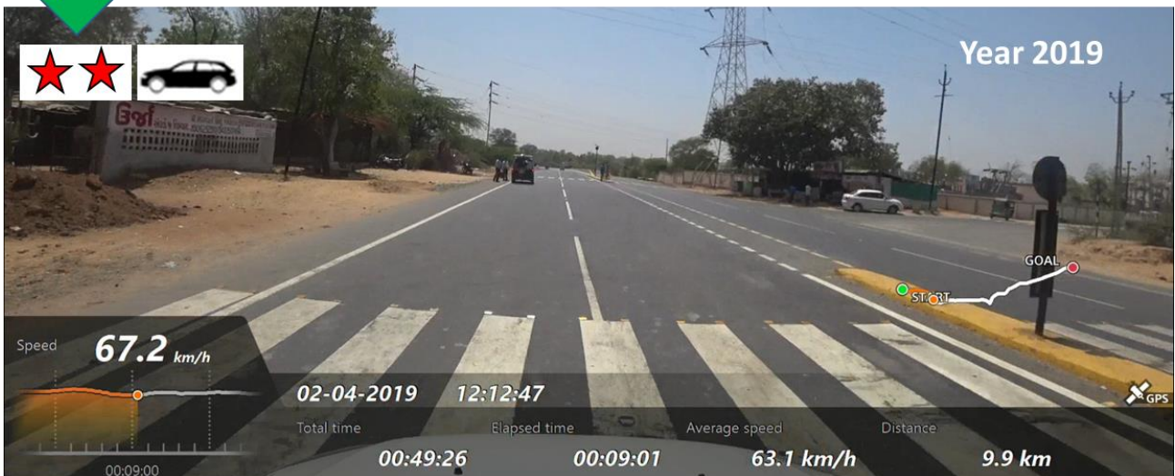
Figure 14 Before and after improvement image of intersection, Km 119.3
