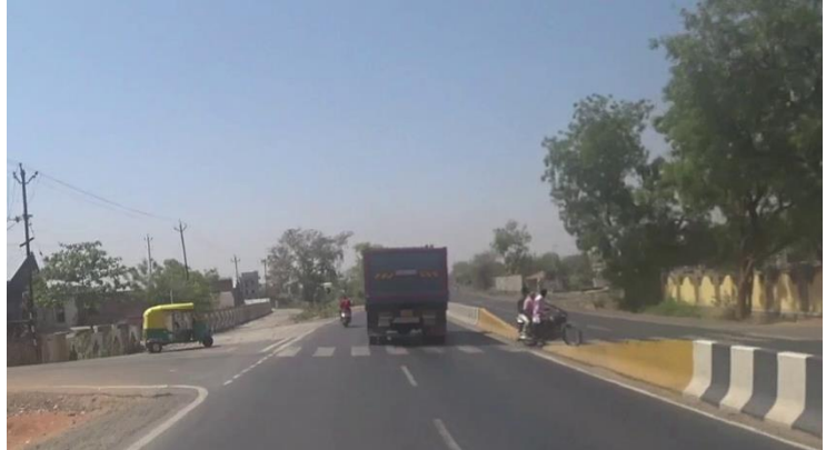
Narrow median width is hazardous for vehicles taking turn. The motorcyclist waiting in the median may hit by any vehicle from the rear or side.
