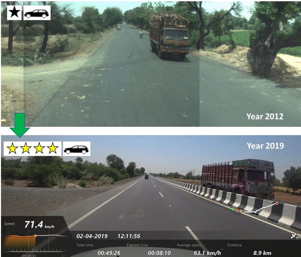
Figure 11 Before and after improvement road image, Km 118.3
