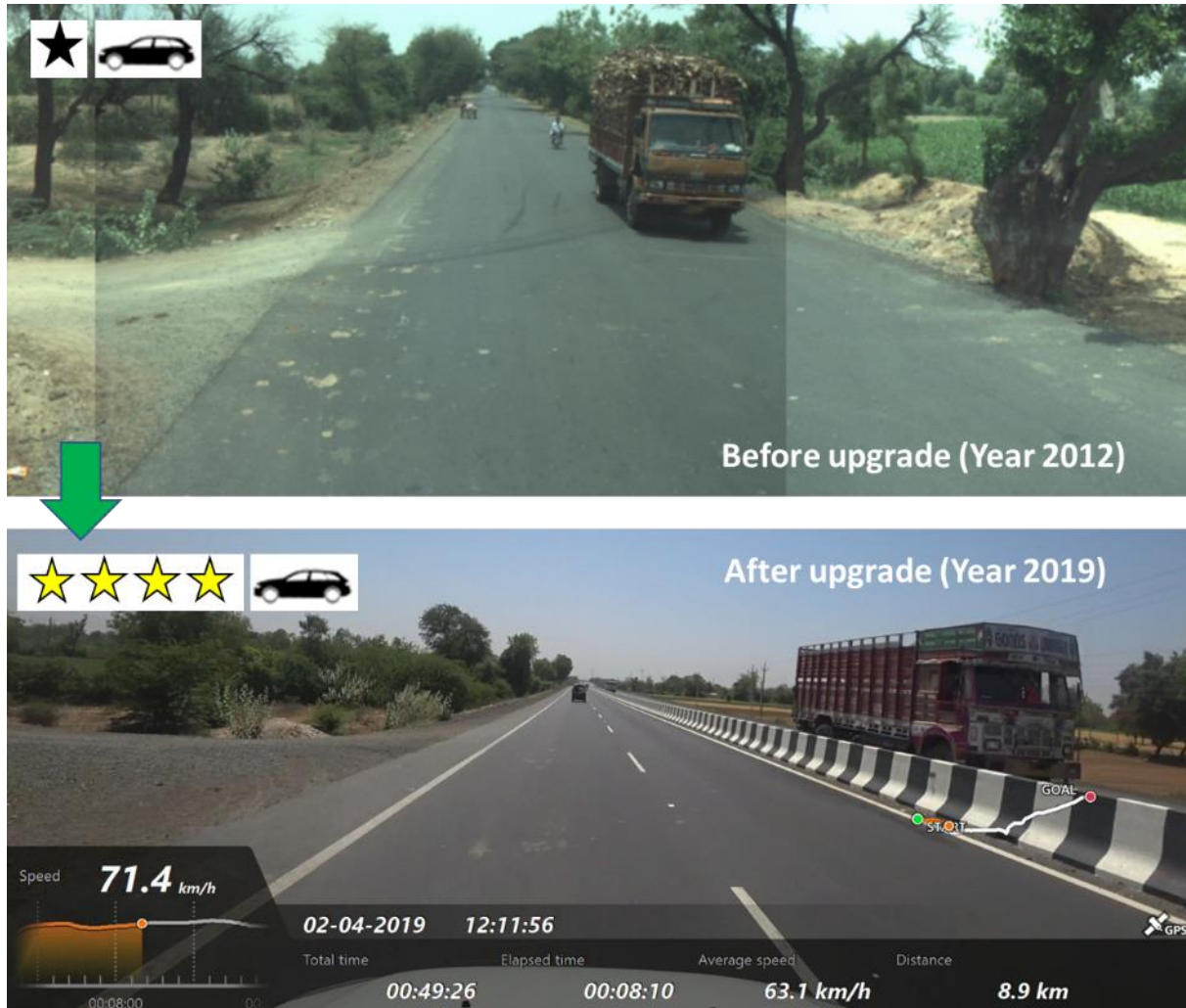
Figure 20: Baseline and post-construction images, Km 118.3 on the Mehsana–Himmatnagar (SH-55) corridor in Gujarat
