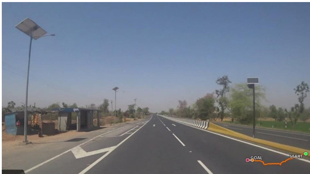
Figure 15: Example of Streetlight and delineation (road markings and signs) on the Mehsana–Himmatnagar (SH-55) corridor in Gujarat
