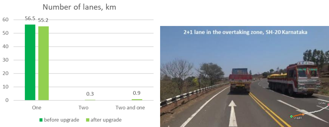
Figure 11: Additional lanes on the Belgaum–Yaragatti (SH-20) corridor in Karnataka
