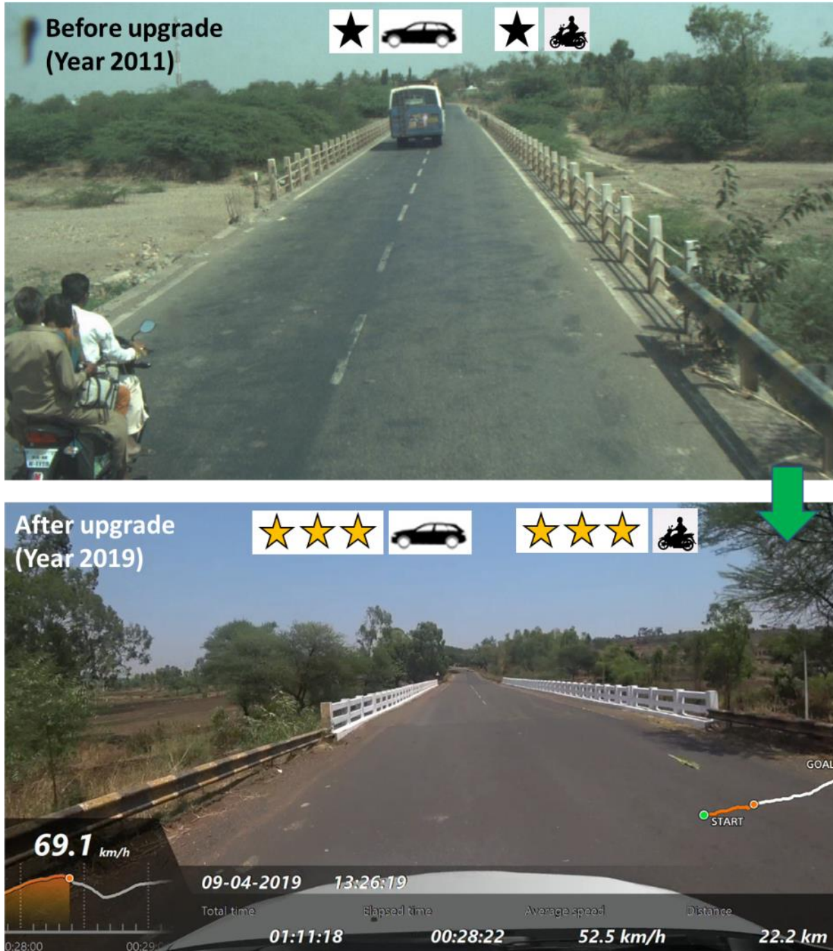
Figure 16 Baseline and post-construction image, Km 22.2 on the Belgaum–Yaragatti (SH-20) corridor in Karnataka
