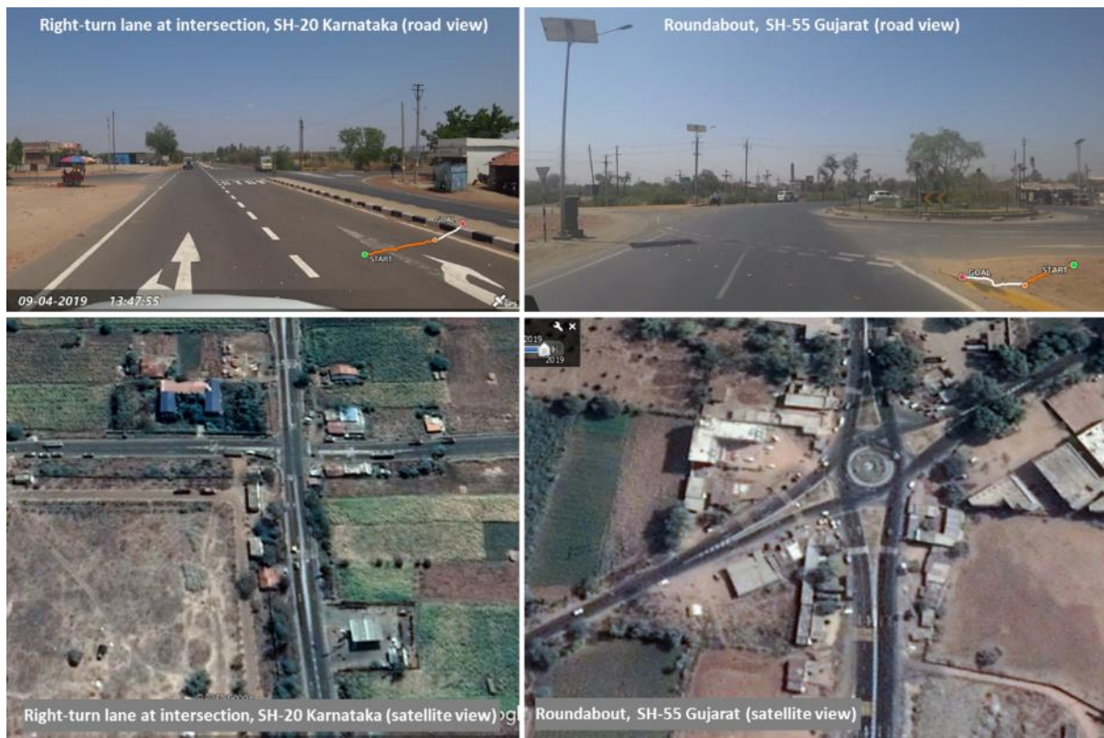
Figure 9: Intersection with turn-lane on the Belgaum–Yaragatti (SH-20) corridor in Karnataka and a roundabout on the Mehsana–Himmatnagar (SH-55) corridor in Gujarat
