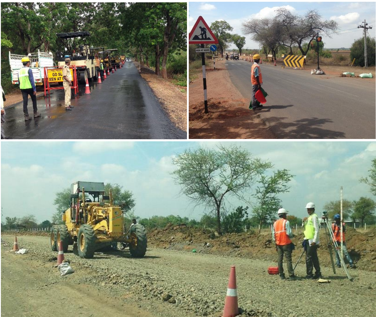
Figure 12 Construction phase, Gujarat India
