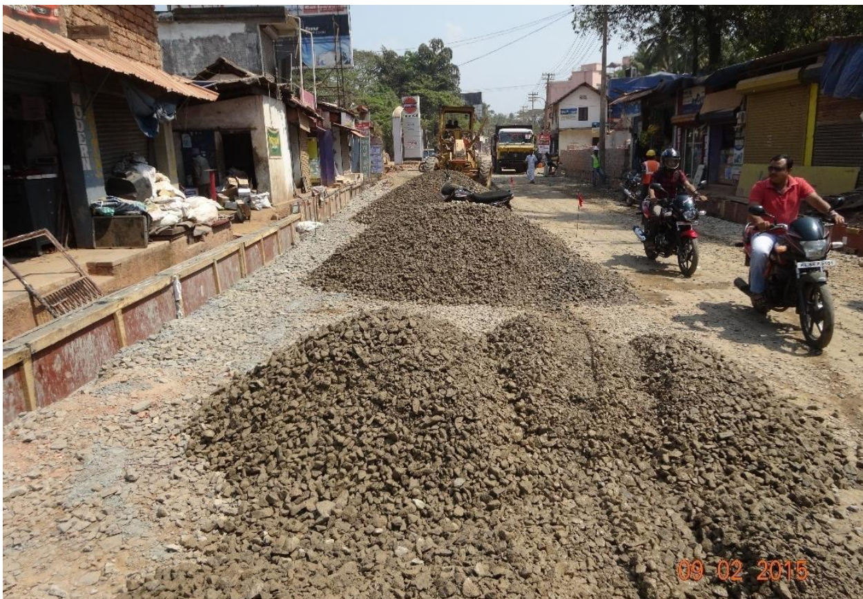
Figure 11 Laying the road base (WMM), Thalassery to Valavupara, Kerala
